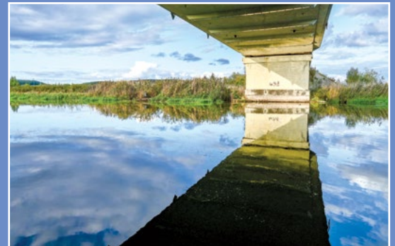
Most na Noteci Netzebrücke
