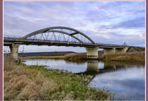
Most na Noteci Netzebrücke
